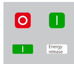
Circuit breaker switched on and no energy storage
